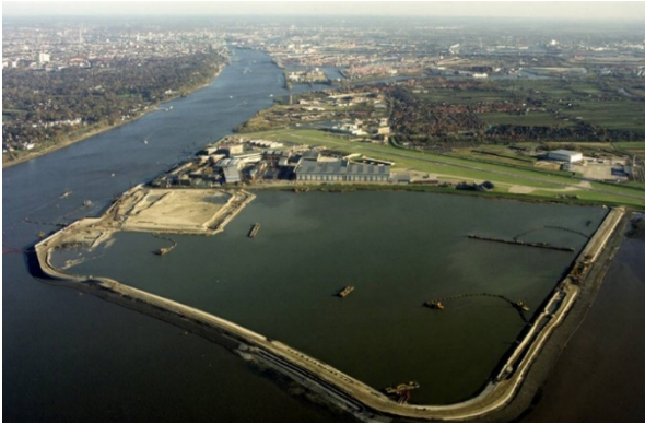
Figure 4.10 Start of the plant extension (ReGe 2021)
