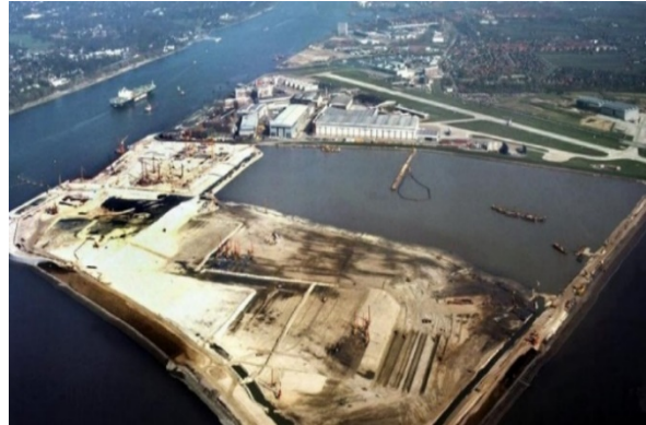
Figure 4.11 Progression of the plant extension construction (Airbus 2002)
