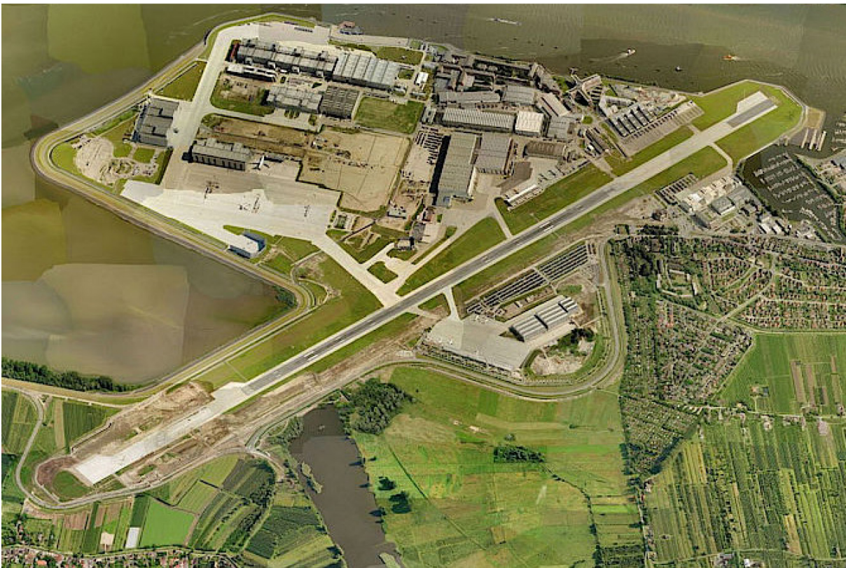
Figure 4.16 Finished plant extension into Mühlenberger Loch and Neuenfelde (Picture from Google Maps)
