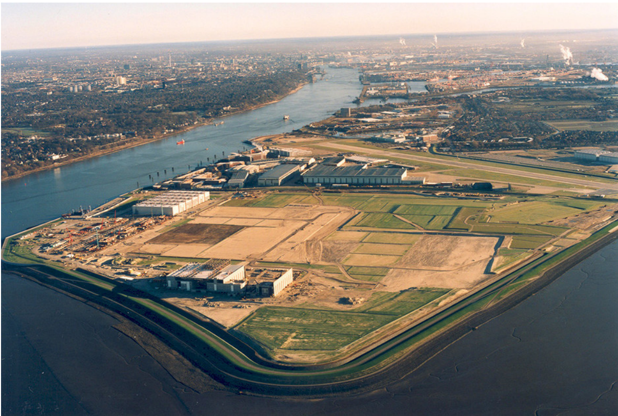
Figure 4.12 Finished plant extension in the Mühlenberger Loch (ReGe 2021)
